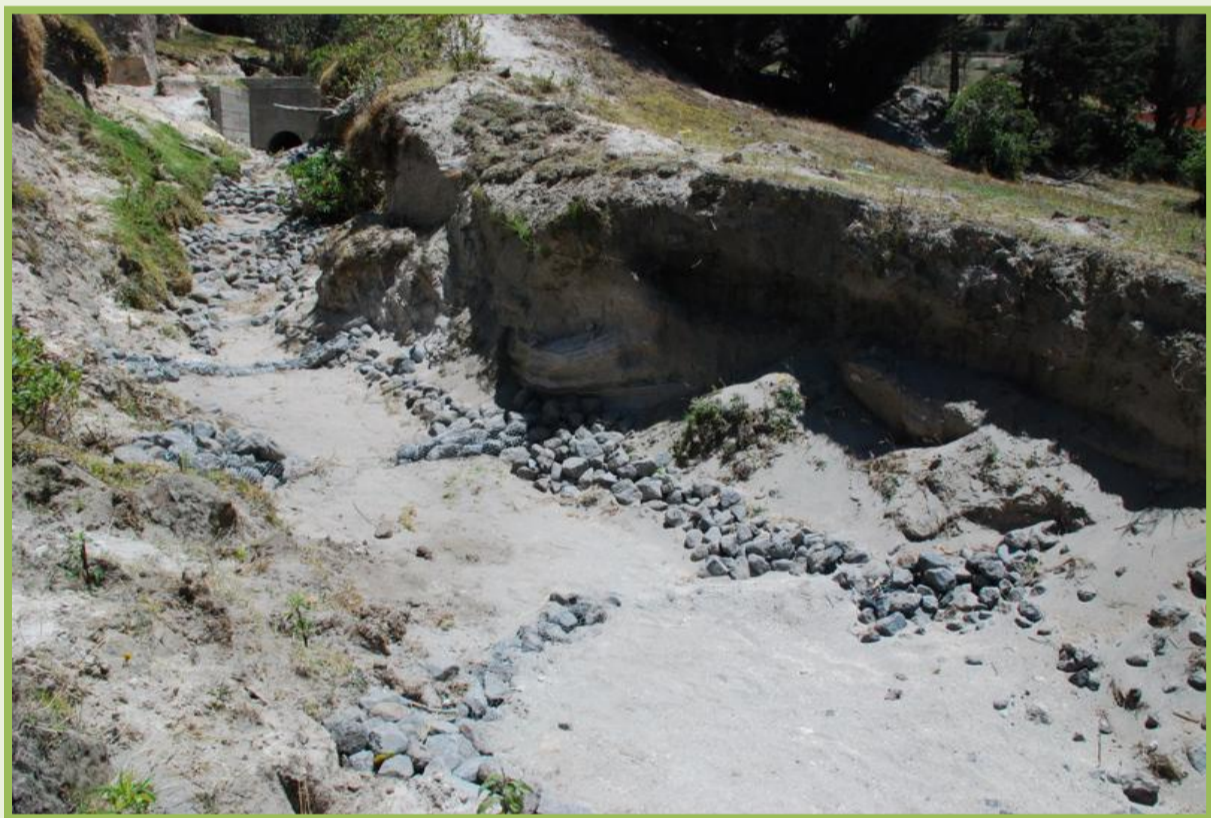
2012 - Alcantarizado de Malingua, post-project. Boulder plunge pools and cross-vanes installed below a road culver outlet to reduce scour and direct stormwater flows away from toe of banks.
