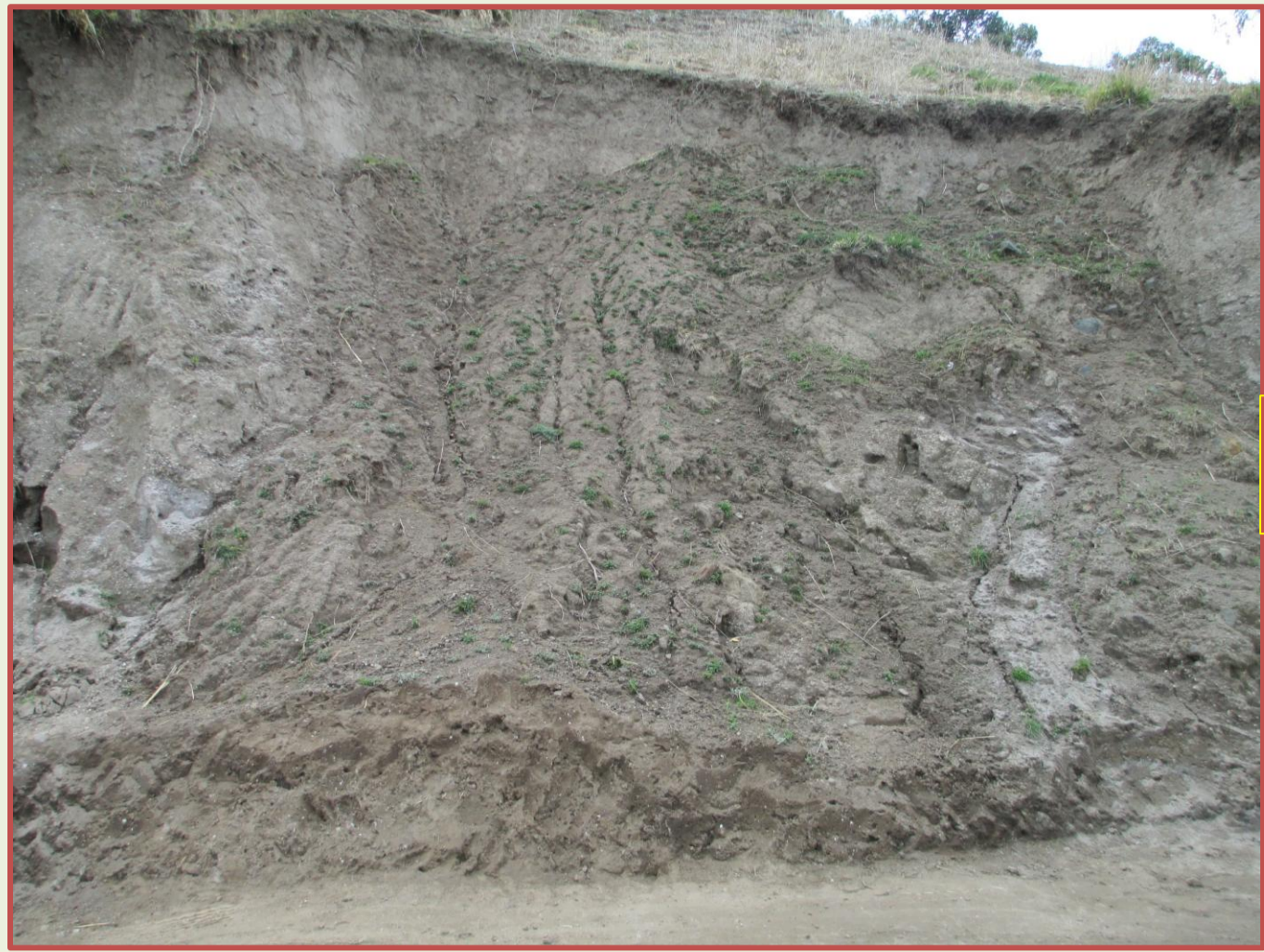
2012 - Chimbusig road cut, pre-project. Slumping of “tierra blanca” volcanic subsoils was causing road closures.
