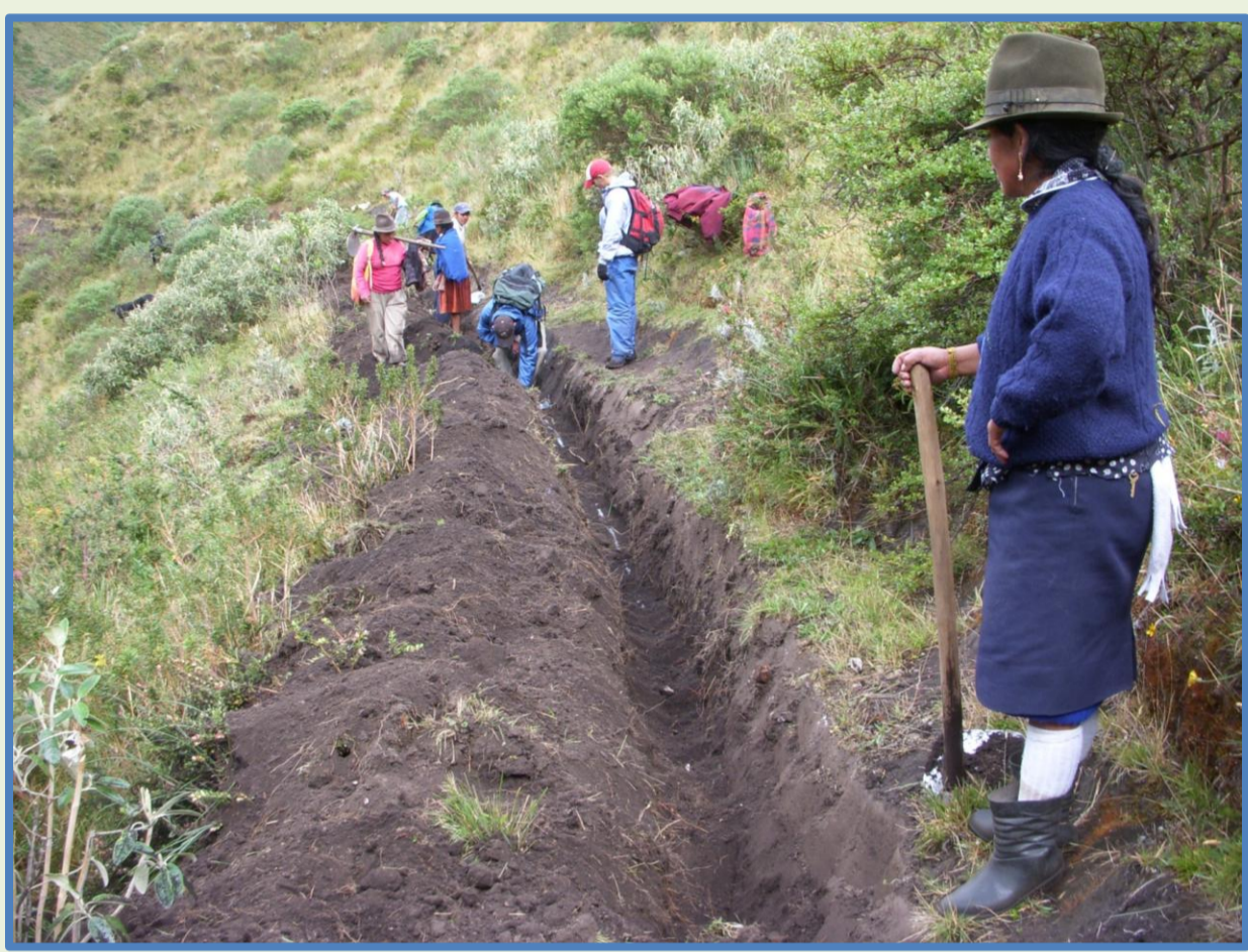
2009, irrigation line from source springs. The minga was digging an improved pipeline through remnant cloud forest “tierra negra” organic soils.
