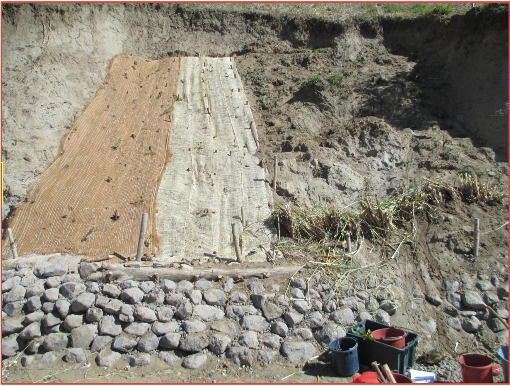
2012 - Chimbusig road cut, post-project. The minga (community work group) and EWB volunteers have installed imported and local erosion matting with native woody species, sigsig grass infiltration hedges, live-stake lechero poles, and boulder toe wall.
