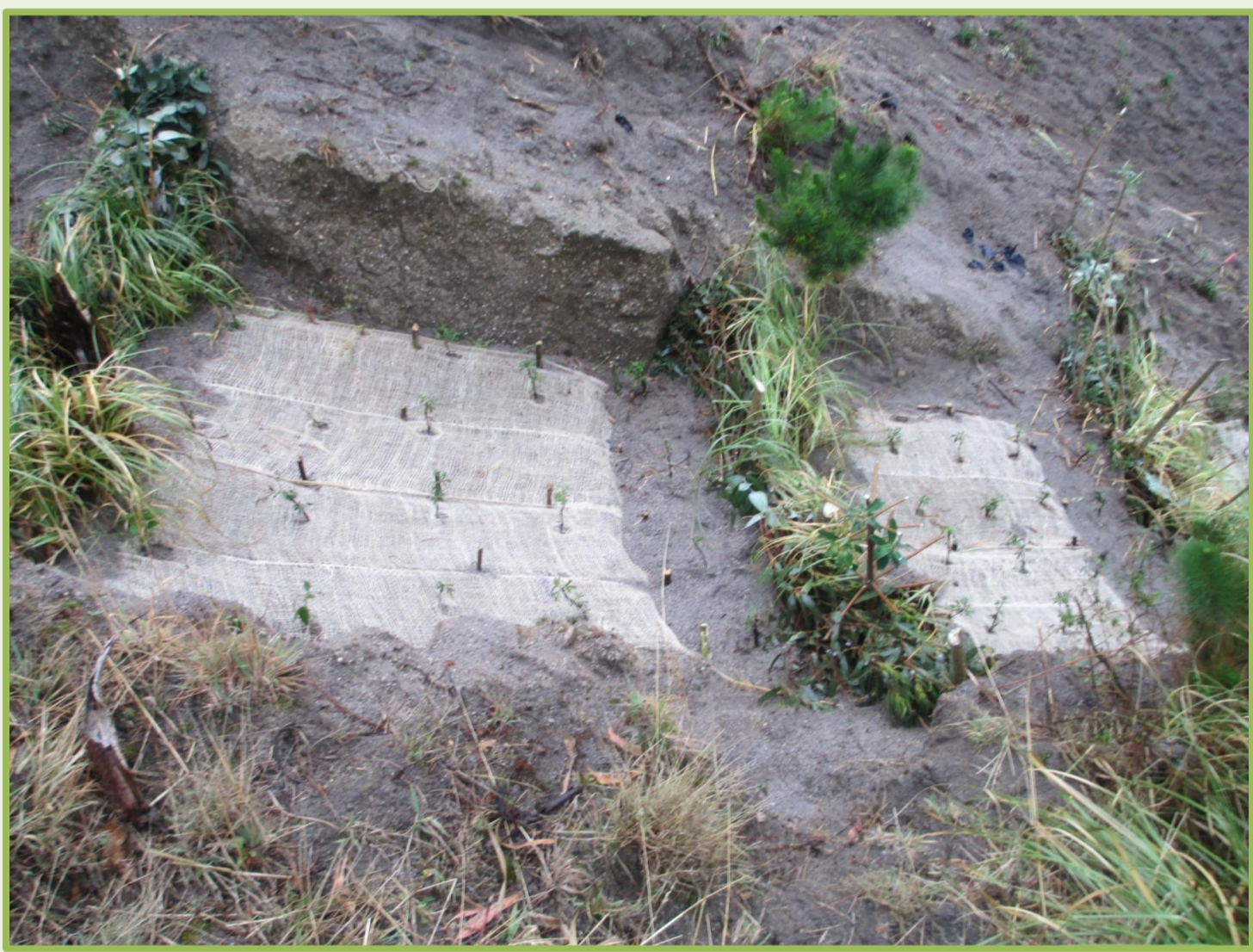
2013 - Erosion gully below pipeline, post-project. Live-stake wicker weirs with sigsig infiltration hedges, local mats, and native plantings stabilized downcutting. Note “tierra blanca” subsoils at the surface.
