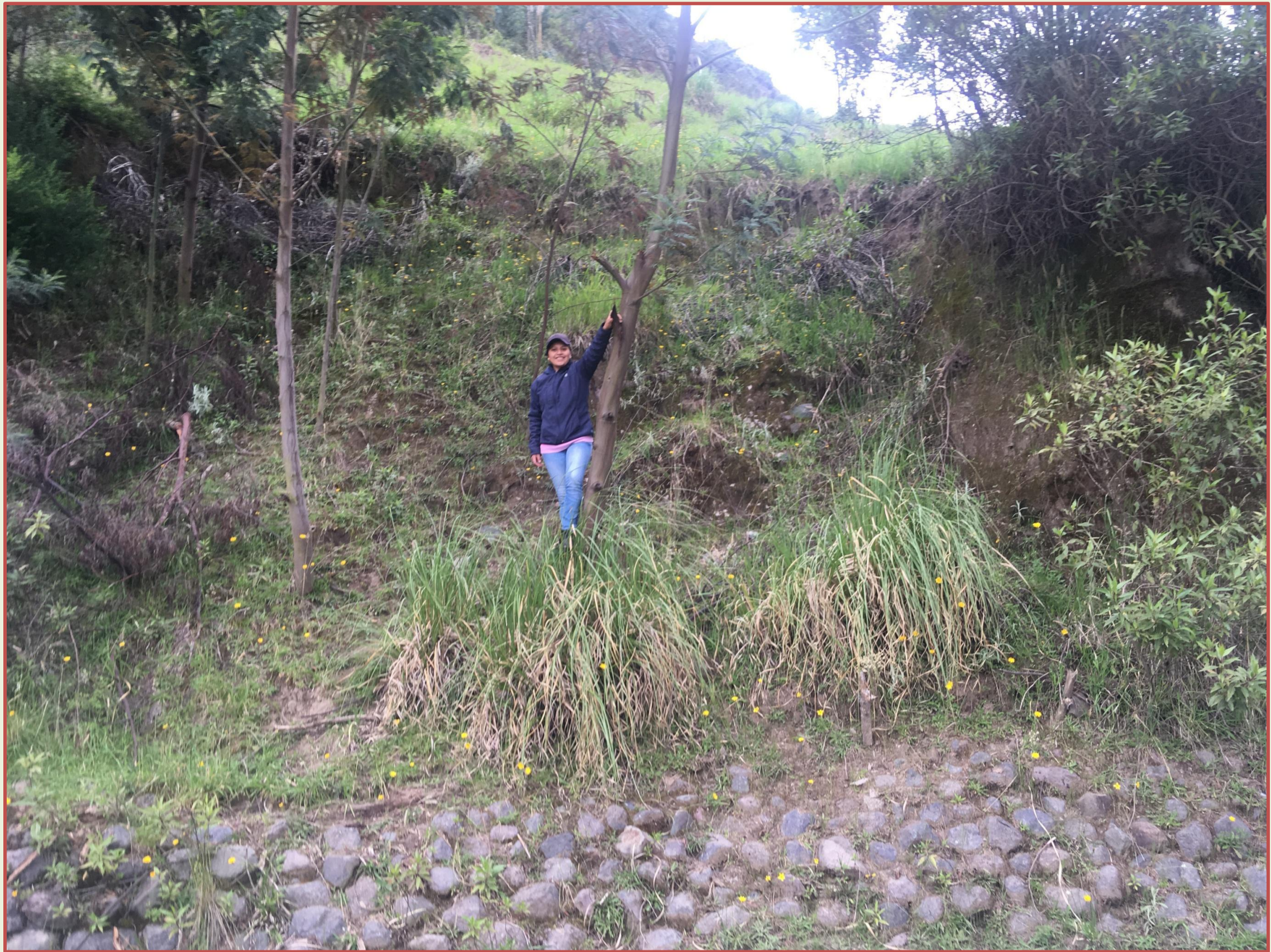
2017 - Chimbusig road cut, 4.5 years post-project, Enma Sacatoro in center of site. The slope now is stabilized by acacia trees over 5 m. tall, vigorous sigsig hedges, boulder toe wall, and many volunteer species.
