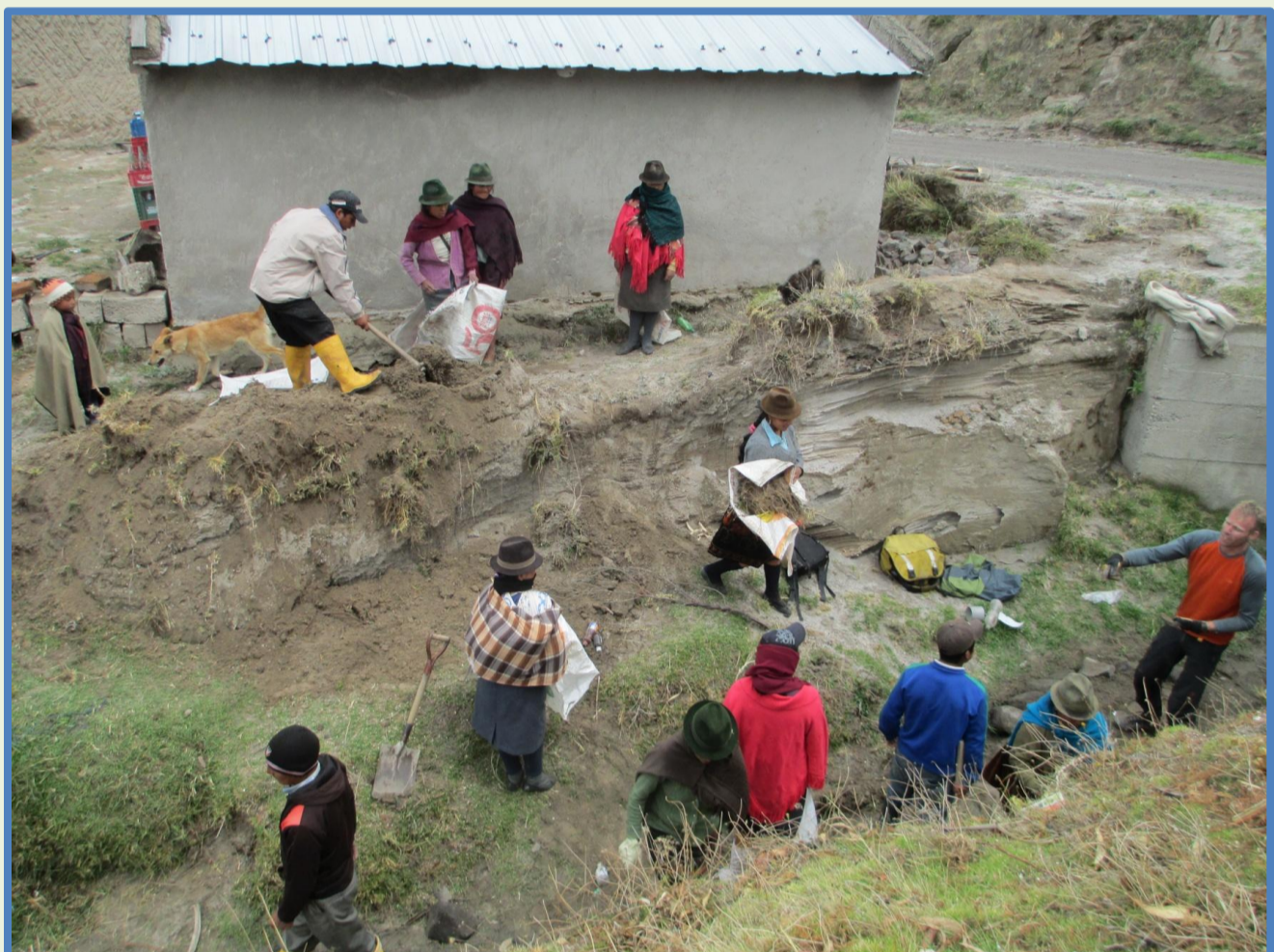
2012 - Alcantarizado de Malingua, project implementation. By installing boulder structures and native plantings in erosion matting, the minga stabilized an eroding storm water runoff channel next to a house.
